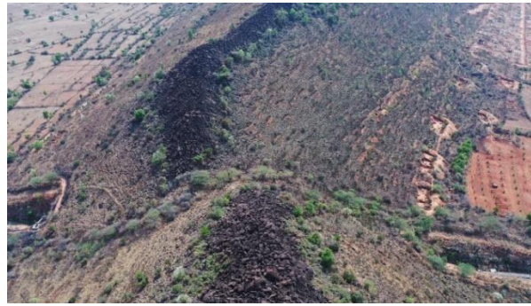
Figure 3. Bird-eye view of the tunnel.
