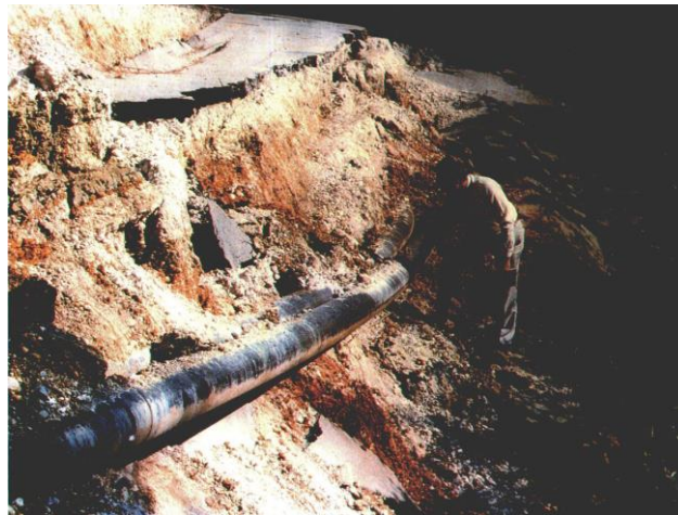
Figure 28. The welded PE pipes stop a road slide [22].
