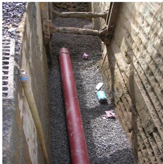
Figure 29. Chippings 4/8 mm (Germ. “Splitt”) as bedding material [24].
