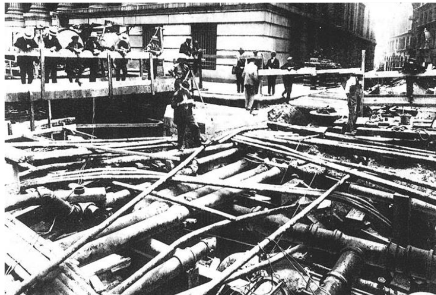
Figure 2. Underground pipes in New York around 1916 [2].
